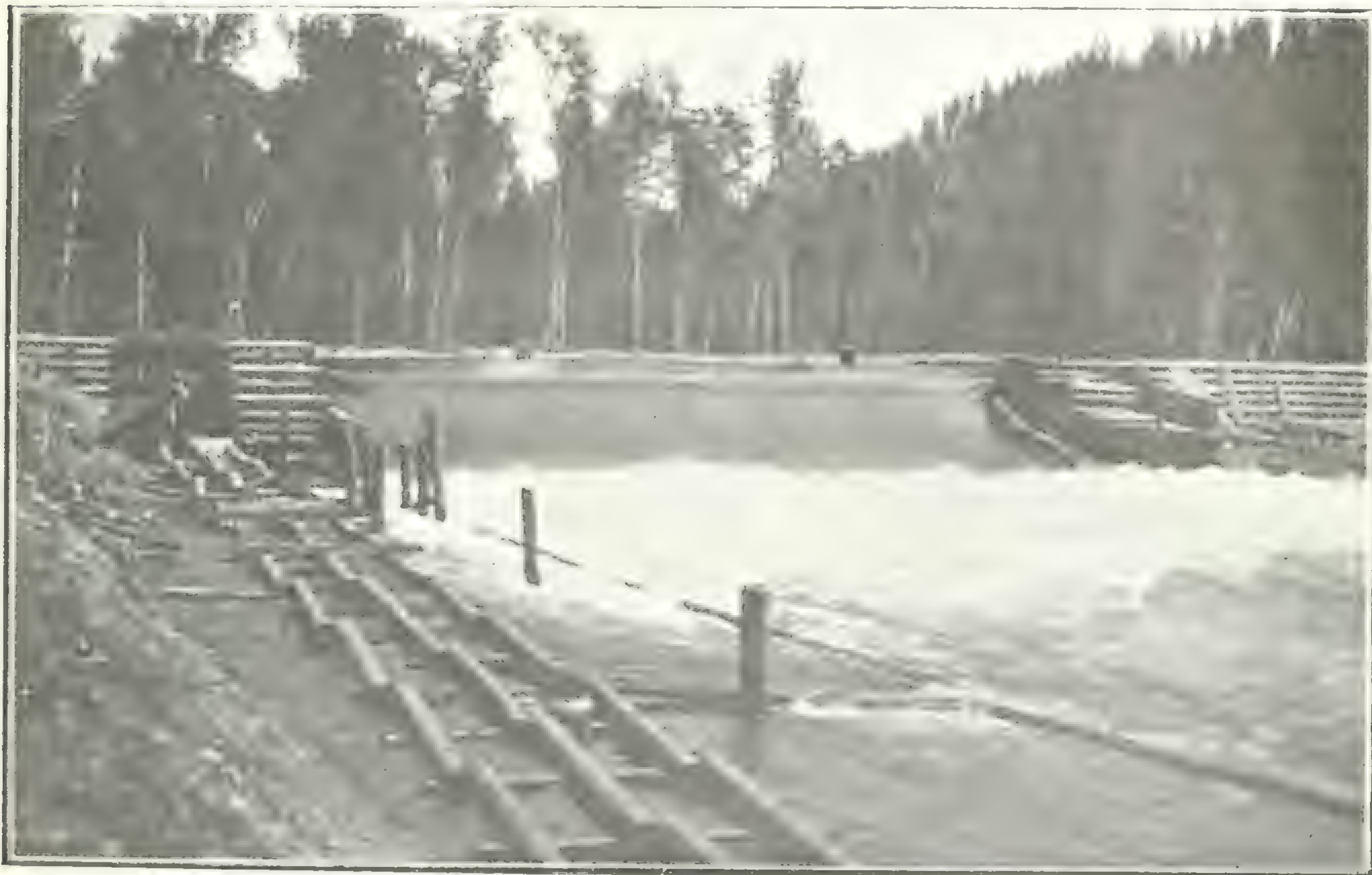
Barricre River Intake Dam City of Kamloops Development.
